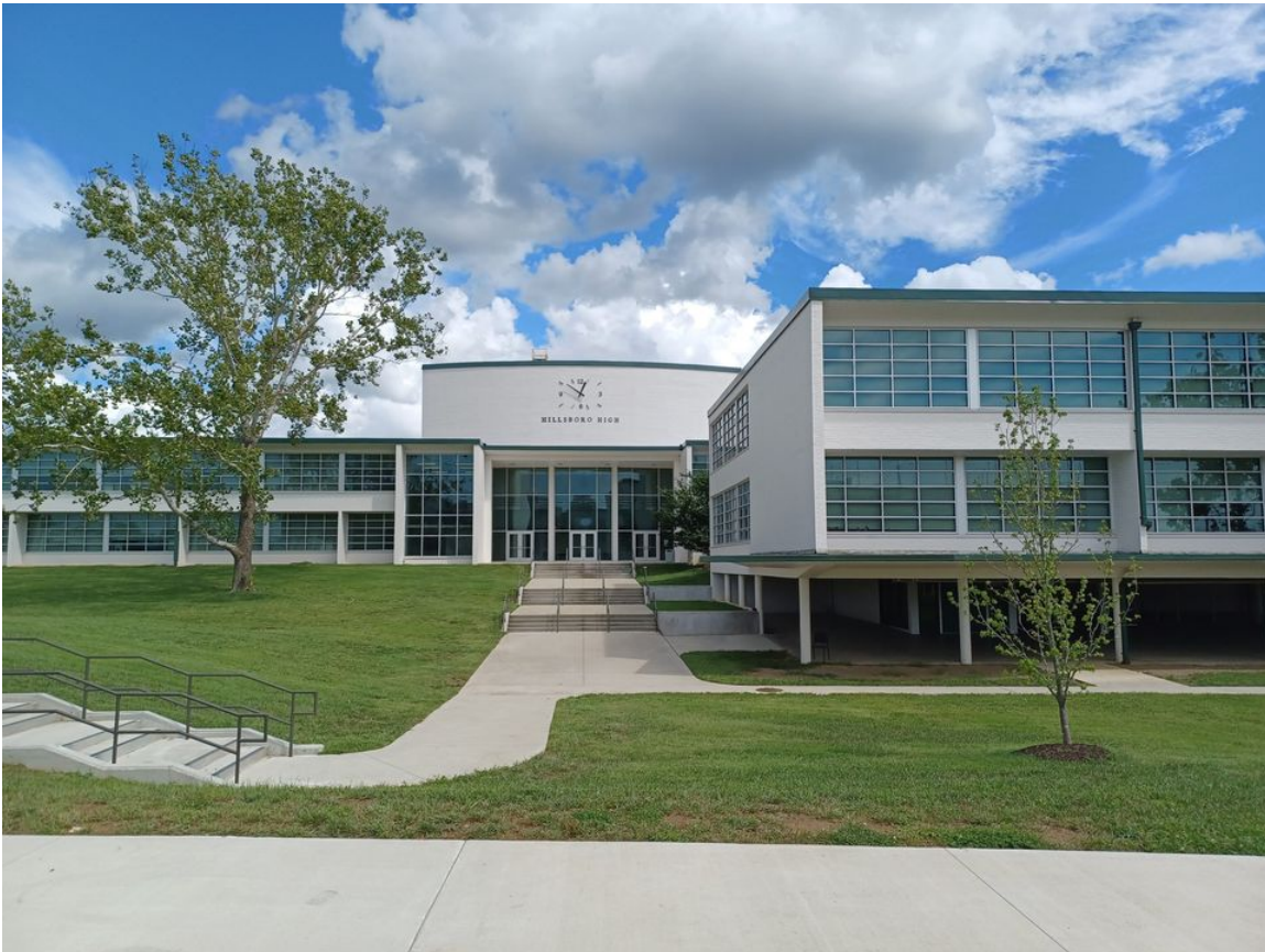
Hillsboro High School recently completed an $88 million full renovation and addition.
